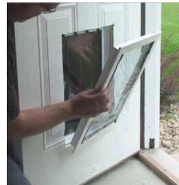
**Step 8:** Using the pre-drilled pilot holes and supplied drill bit, drill and insert one screw. Make sure the door is level. When level, tighten the inserted screw. Affix remaining screws into place using the pilot holes as guides. (*Security Boss Manufacturing has included One-Way Security Screws as well as Philips head screws to give customers a Tamper-proof option in their door installation.*)
