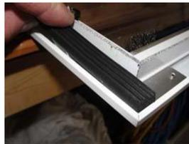
**Step 7:** Put the inner frame (the one with the insulated security panel) into the rough opening in the people door. Snap the outside frame into MaxSeal door and sleeve the pet door frame together.
